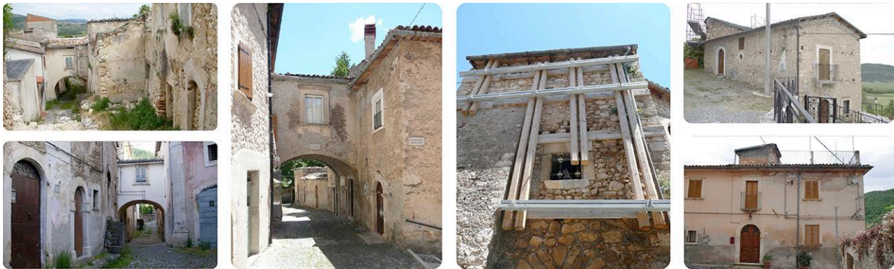
Figure 1. Views of the medieval village of Caporciano. The aggregate consists of approximately 300 buildings, with its traditional architecture of rural type, consisting mainly of vertical walls (coinciding with the elevated structure) in local stone, with rustication and gravel of various sizes, which can reach 90-100 cm thick, even with small-recovered brick elements. The village has an outer belt of expansion characterized by newer buildings (from the 50s onwards), with concrete-frame technology and plugging in semi-solid blocks of brick or masonry bearing.
